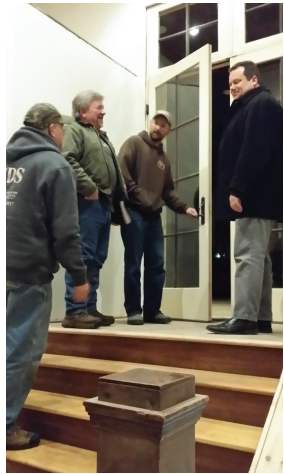
Banks Township Trustee Tom Cooper and Supervisor Thomas Mann check out perfect hardwood stairs recently uncovered during renovations and new doors that open into the hall's banquet room.
